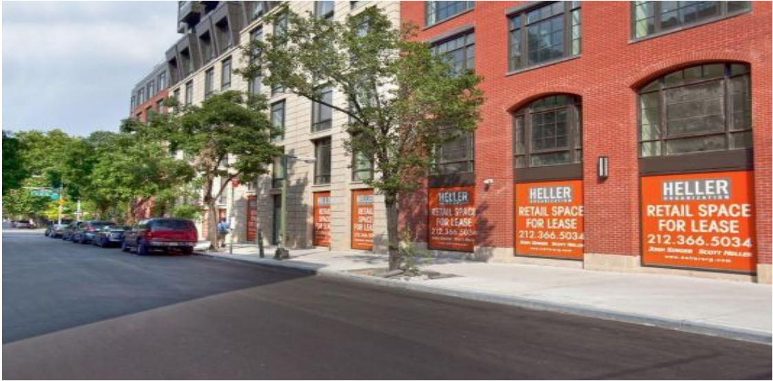
Blockfront of Bedford Avenue, between North 11 th & North 12 th Streets
