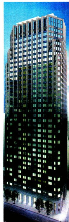
75 Wall has a beach on its roof.
